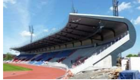
INDUSTRIAL, SPORTS AND OTHER STRUCTURES
